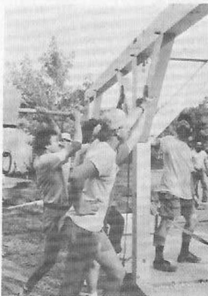
Timber framing students and staff of Upper Loft Design, Inc. are pictured at work erecting an Alpine farmhouse frame at a recent week-long workshop in Clayton, GA. Owner John Koenig will teach a weekend seminar on timber framing at Highland Hardware September 15-16. His article on the subject of timber framing appears on page 7.
