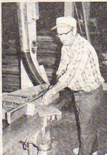
Using the Makita planer/jointer to surface the Cocobolo shoe of a long jointer plane.
